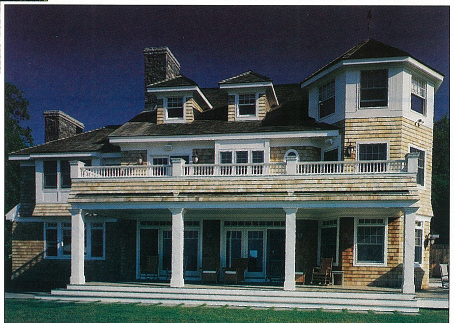
Left: The kitchen features "Wood-Mode" cabinets, granite countertops, limestone floors, and modern appliances. Right: The view of the house from the terraced yard, which looks onto the pond.
