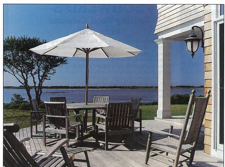
Ipe decking on the porch has weathered to a lovely grey.
