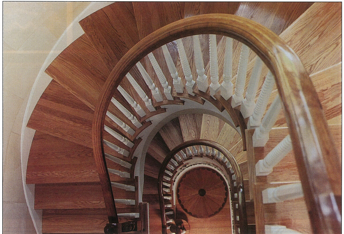
The grand staircase leads down three floors to a laser-cut medallion on the first floor. Woods used here included cherry, walnut, and red oak.
